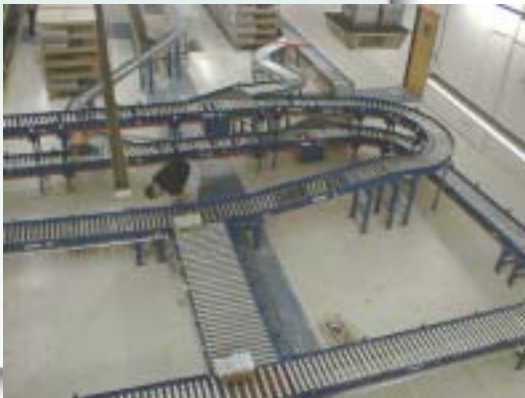
Presort System with sorting machines at top and outgoing conveyors at center.
