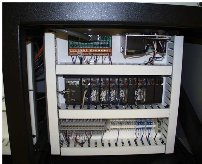
At Station 5: Oven Loader Controller with Think & Do WinPLC (at left center)
